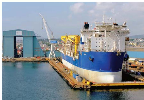
Norway: Alvheim FPSO topsides installation, Haugesund
