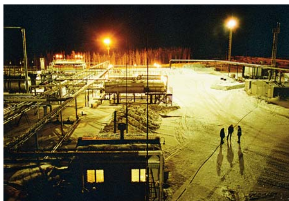
Russia: Sothemyu-Talyu field facilities located in the Komi Republic
