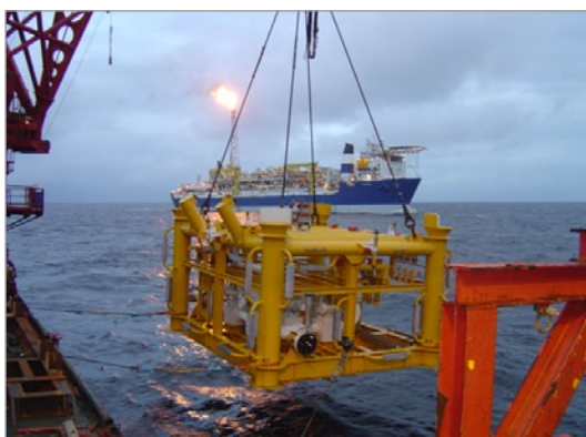
VOLUND SUBSEA INSTALLATION & ALVHEIM FPSO, NORWAY
