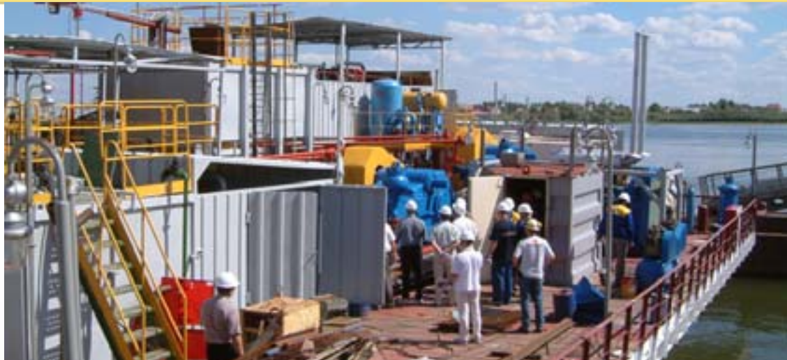
Alterations being made on the mud barge
