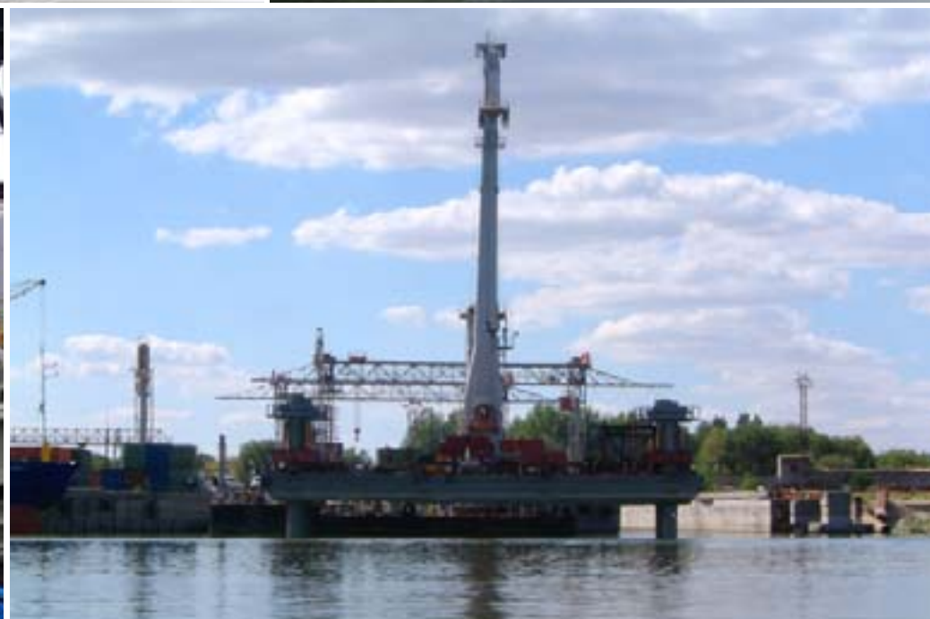
Load testing on drilling rig pontoon
