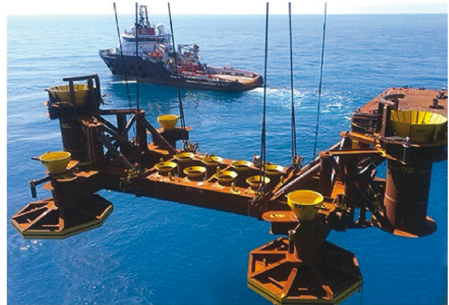
Pre-drilling template installation
