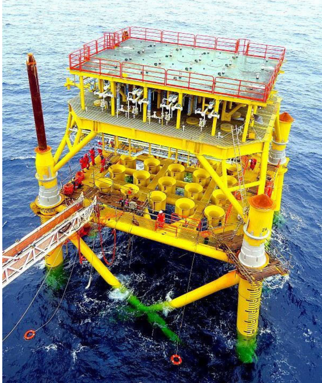
June - Jacket installation
