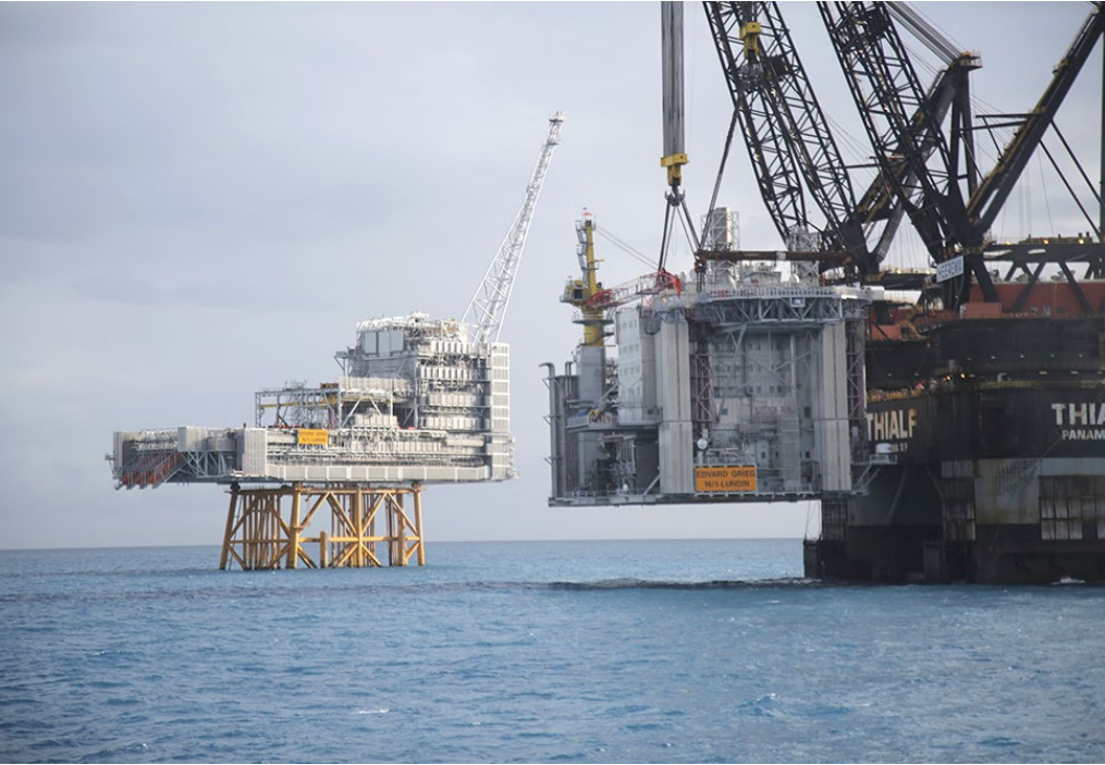
Edvard Grieg topsides installation by heavy lift vessel Thialf
