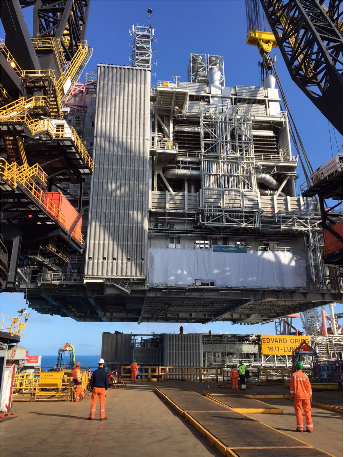
Edvard Grieg topsides installation by heavy lift vessel Thialf
