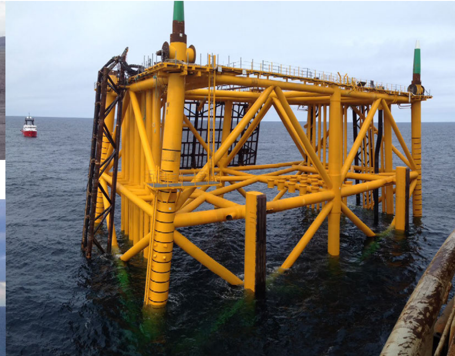
Jacket installed on location, May 4 th
