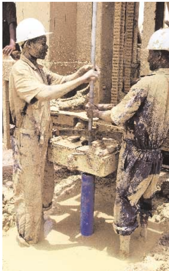
Drilling of water well, sponsored by Lundin Sudan Limited.
