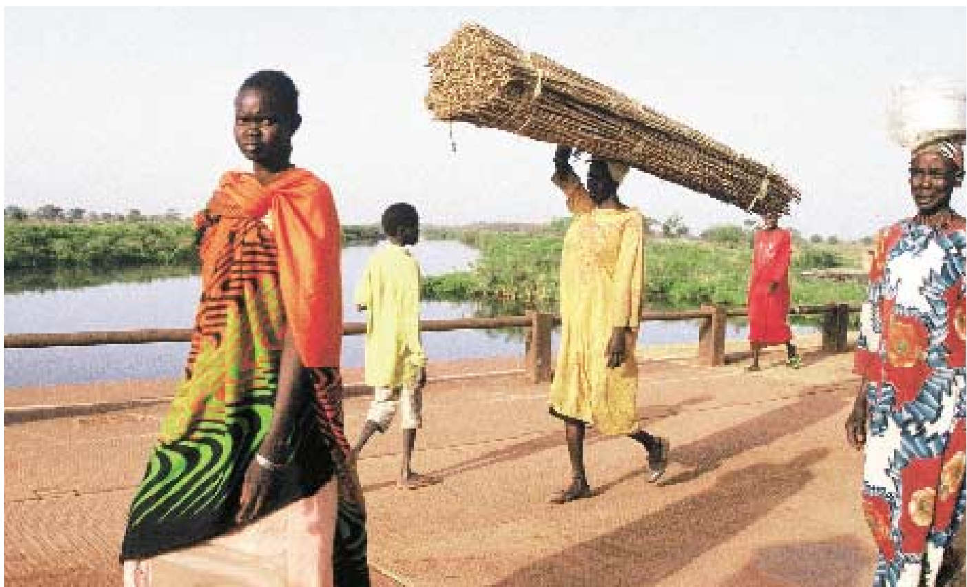
Bridge built by Lundin Sudan Limited over the Bahr el Ghazal river in Southern Sudan
