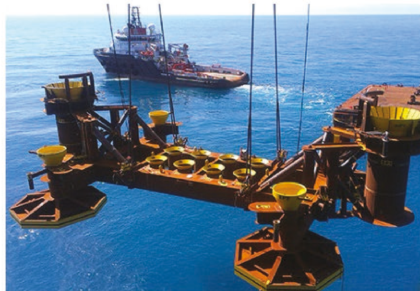
Pre-drilling template installation
