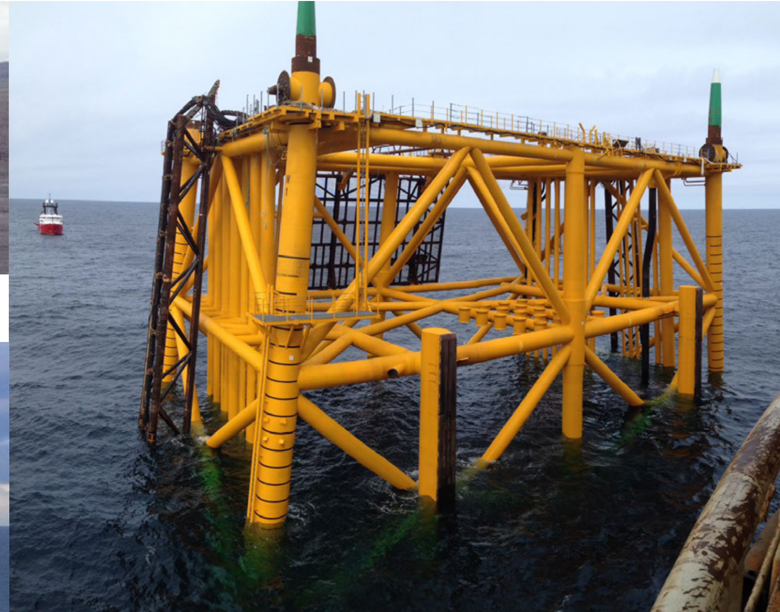
Jacket installed on location, May 4 th
