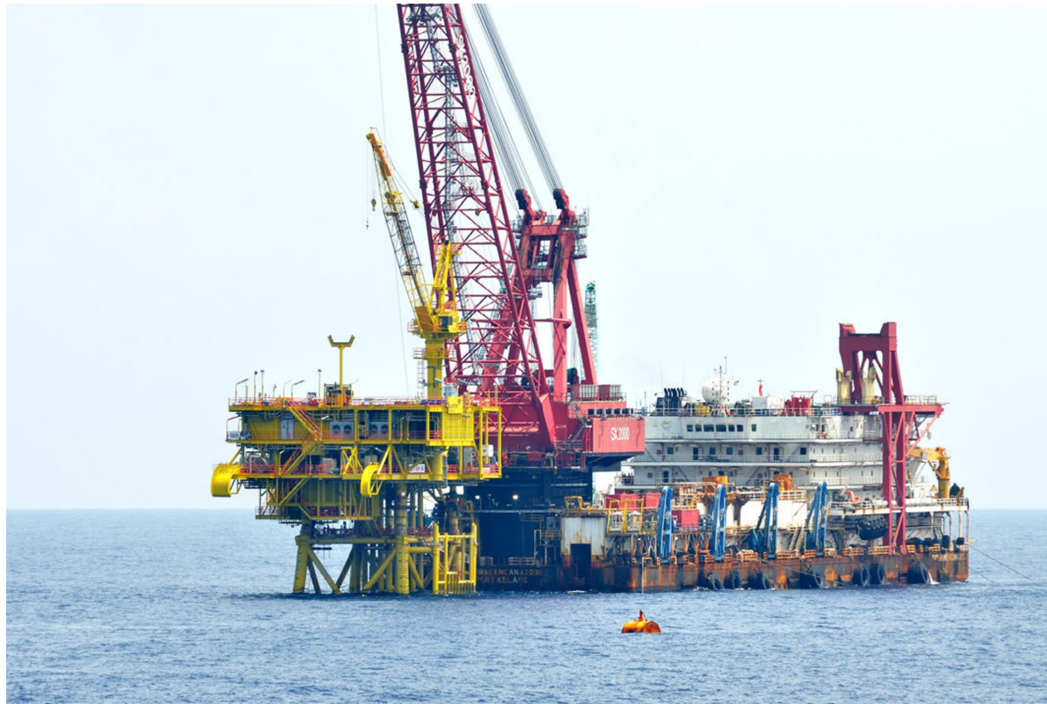
October - Installation of the Bertam Wellhead Platform
