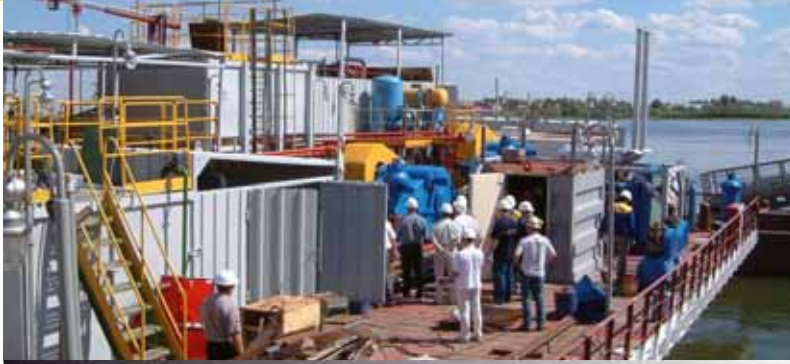
Alterations being made on the mud barge
