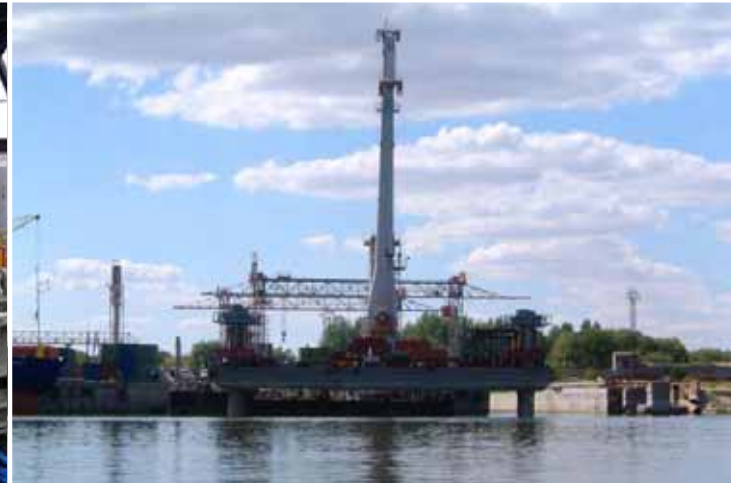
Load testing on drilling rig pontoon
