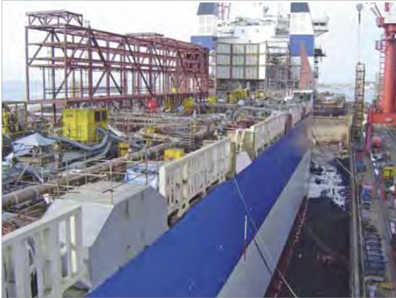
Alvheim FPSO modifications at the Keppel shipyard, Singapore
