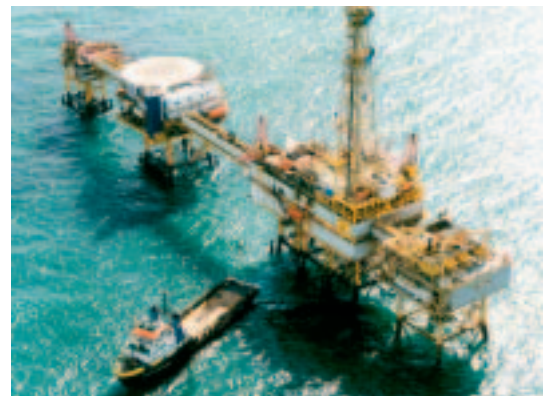
L7 CENTRAL PROCESSING PLATFORM, NETHERLANDS
