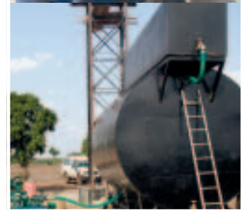
PHOTO SEQUENCE FRESHWATER FILTRATION UNIT INSTALLATION
