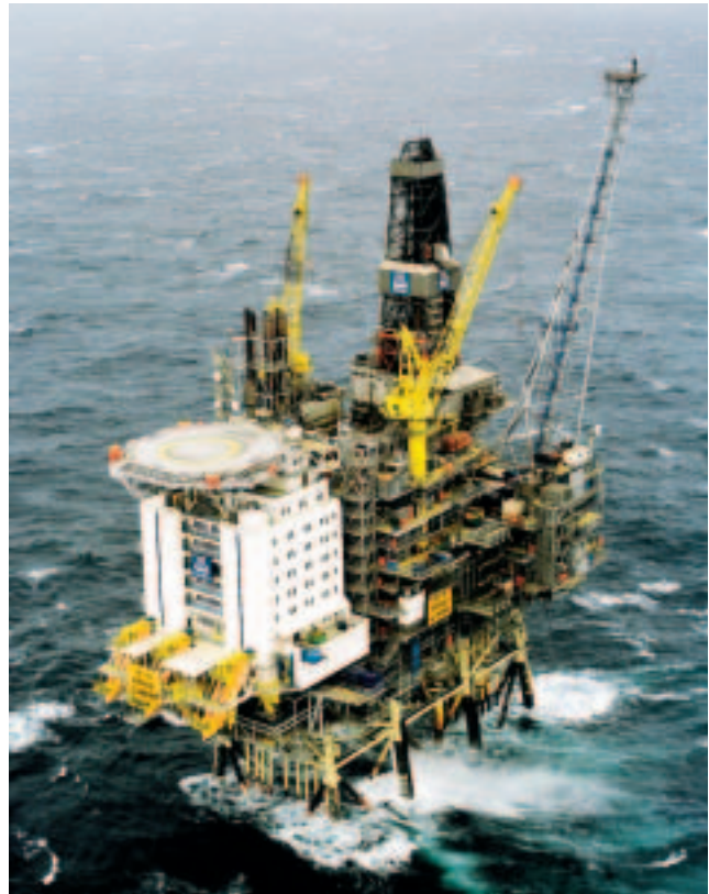
BRAGE PLATFORM, NORWAY
