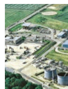
Production center Villeperdue
