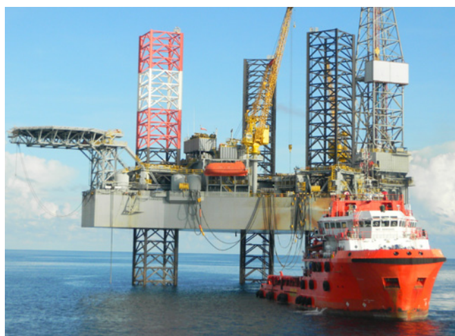
Malaysia: Drilling operations
